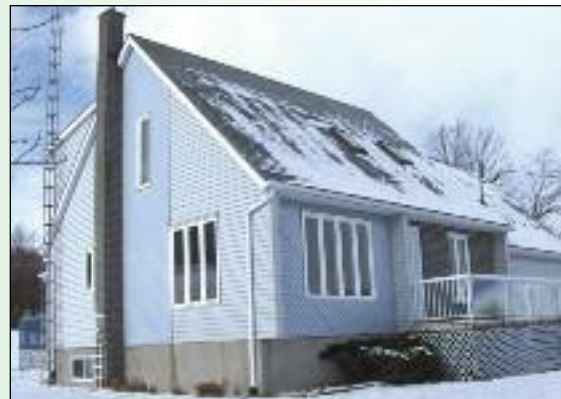
Before renovation in Dunham
