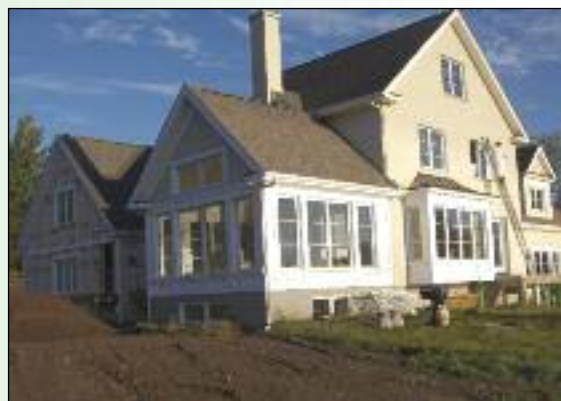
After renovation in Dunham
