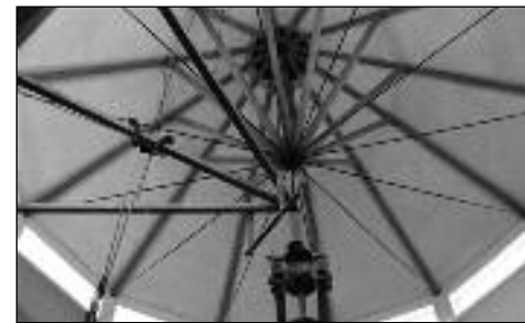
Image of ceiling in Walbridge barn.
